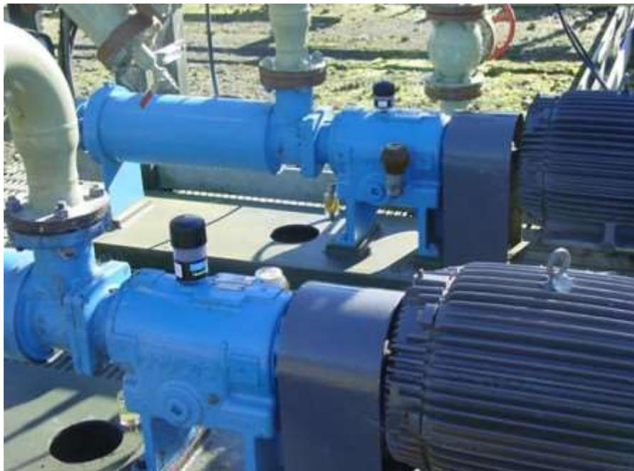
With all moving and revolving parts, Gearboxes are extremely vulnerable to malfunctions if contaminated or improperly lubricated. This means that contaminants can not only cause a breakdown in the health of the lubricant (and thus a failure in the lubricant's ability to perform efficiently) but will also interact with the moving surfaces to cause wear, leading to component failure.
